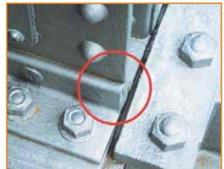
Spilt Steel Grit gets into every nook and cranny of a surface.
